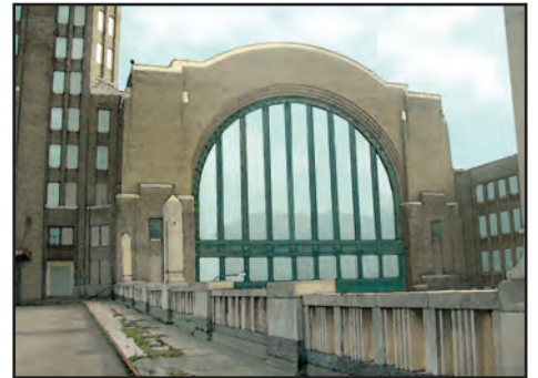
SEPTEMBER (Central Train Terminal)
